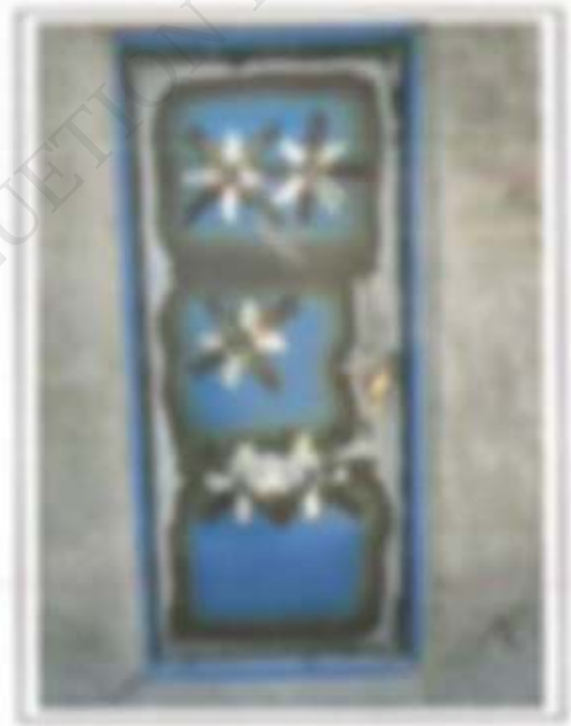
Photograph 5. Photograph of unexposed side of door after the test
